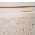
After fitted any excess silicone that squeezes up is removed
